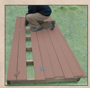
The old fashion way - Using a screw gun and screws means sore knees and in 3 minutes time installing only 2 deck boards.
